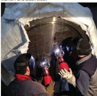
In tube to tube sheet applications, preparation is a very important aspect to guarantee repeatable and quality welding results. The following steps are discussed at each project and are essential to ensure the success of your process:
